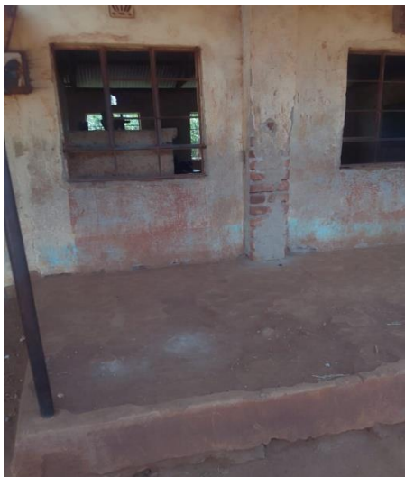
Condition of the classrooms.
