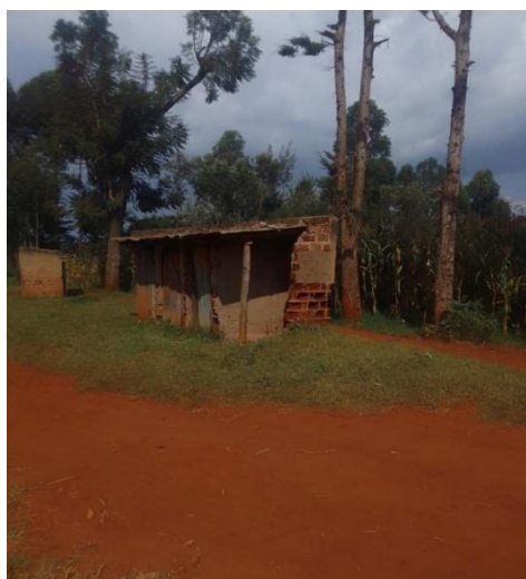
Condition of the toilets
